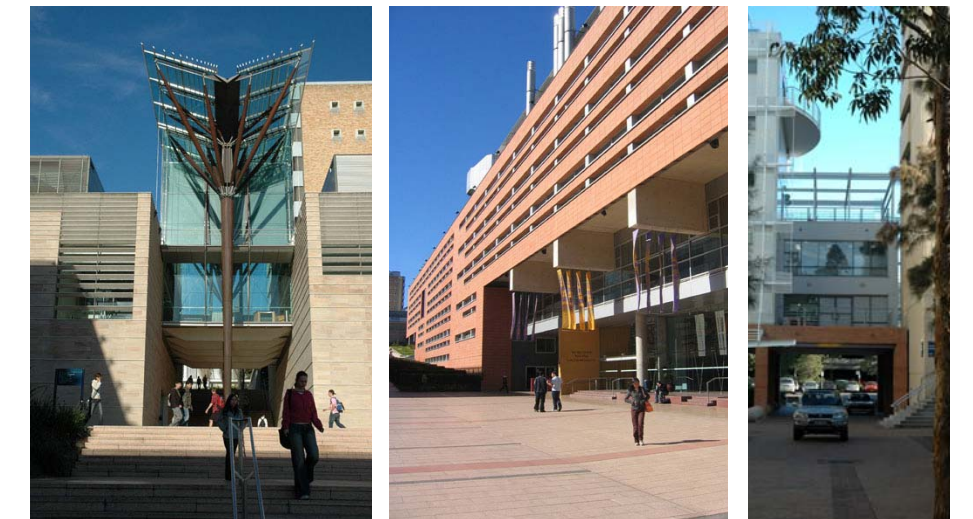
The Red Centre's through building links engage Science Square which informs ground floor wall alignments. The relationship to Science Square is interpreted in the composition of large openings in the building's north elevation. At ground level the links also connect with a courtyard and service lane of the Main Building.
