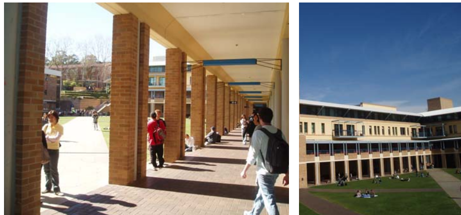
The colonnade of the Quadrangle building expands the extent of the central space at ground level, provides sun and rain protection, and fosters pedestrian amenity. Irregular alignments on the inside of the colonnade, excessive depth and obstructions within the space can detract from the function and potential clarity of such a space.
