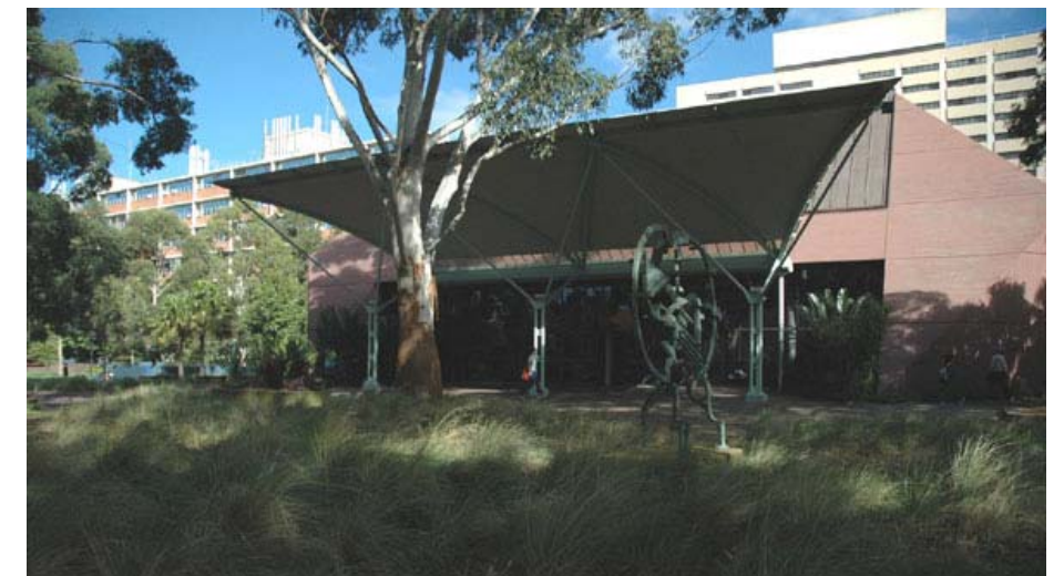
The Sir John Clancy Auditorium and independent canopy structure successfully addresses Chancellery Forecourt, otherwise it is a generally weak building in the round.
