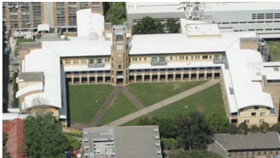
The Quadrangle Building is strategically located at a campus cross roads linking University Walk to High Street and Barker Street, and has a purposeful relationship with connective campus spaces. The courtyard accommodates diagonal movement through the campus, an attribute shared by several campus gathering spaces.
