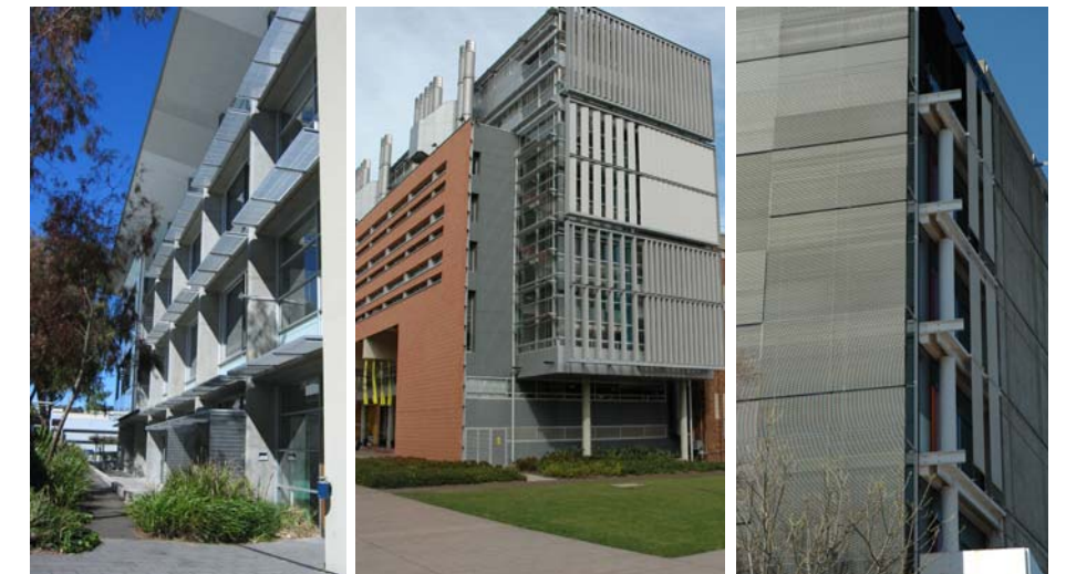
The Red Centre is an example of both passive and active sustainable strategies in practice. The thermal flues actively draw air through the building, ventilating the rooms while expelling warm air. Both the building's strategic orientation to north and its minimal depth allow a high percentage of natural day lighting. Other passive sustainable principles include the protection of west facing glass panels with operable vertical shading devices as well as the integration of thermal mass in the form of terracotta tiles along the northern façade.
